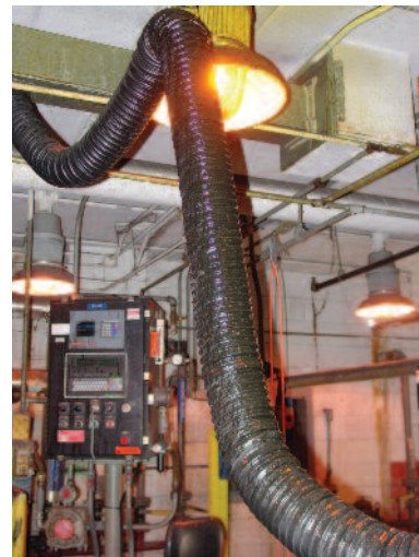
e. Ductwork includes too much flexible hose
